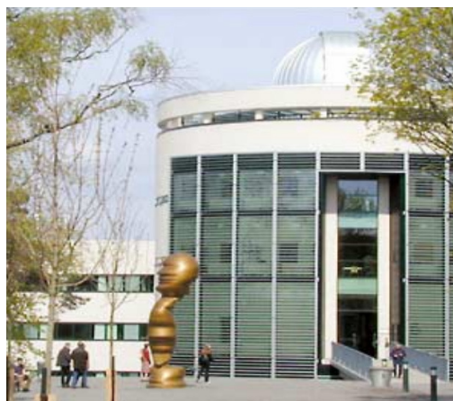
The main entrance of the Albanova University Center, KTH.
